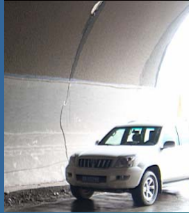
Construction joint offset
