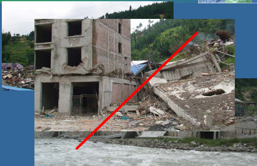
Surface Rupture of the Earthquake Fault
