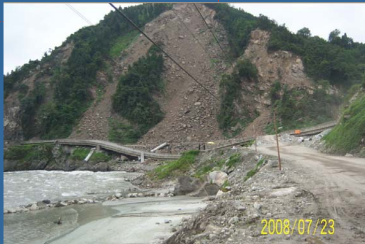
Baihua bridge (after demolition)
