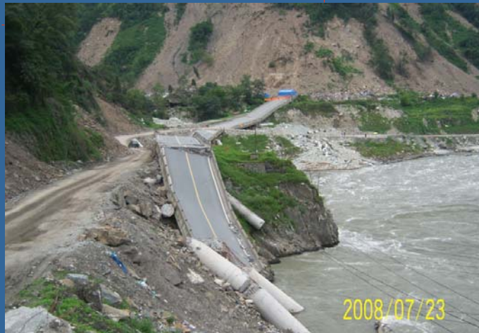
Baihua bridge (after demolition )
