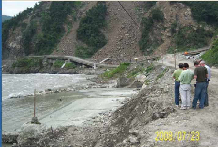
Baihua bridge(after demolished )
