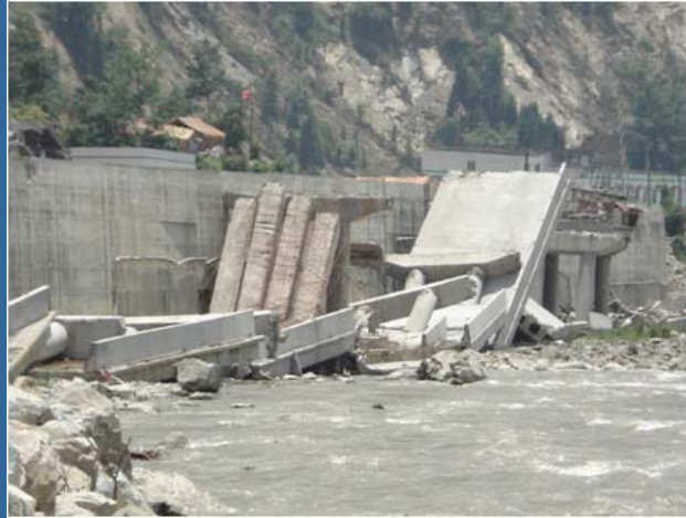
Shunhe bridge totally collapsed in Yingxiu (bridge longitudinal direction was parallel to the fault line)
