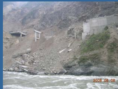
Landslide crushed the bridge on Du-Wen Road
