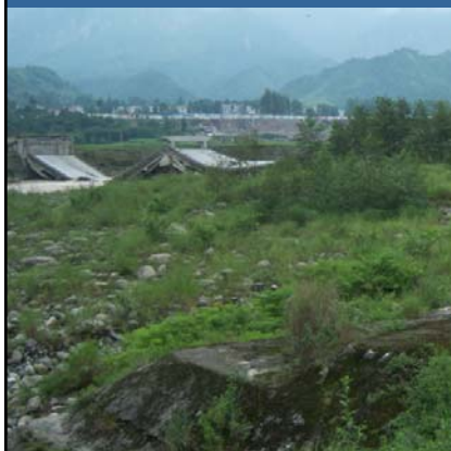
Xiaoyudong bridge (4 spans continuous arch frame)
