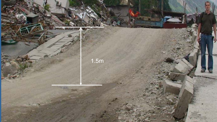
Surface Rupture along the Old Highway near the Collapsed Building
