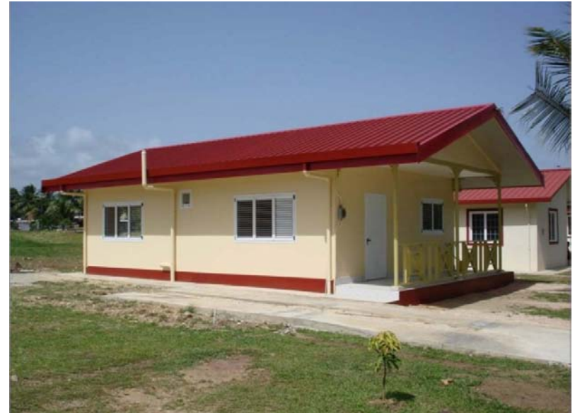
Image w permission Steel Frame Housing USA
