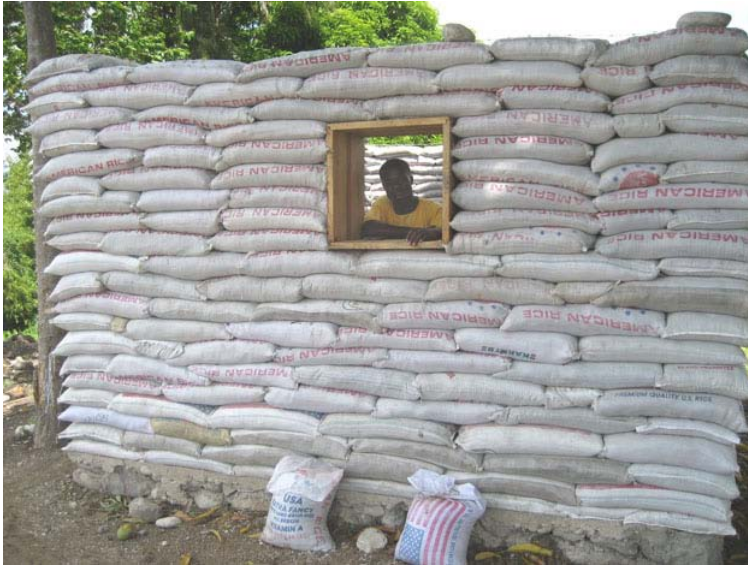
Image used with permission from www.earthbagbuilding.com
