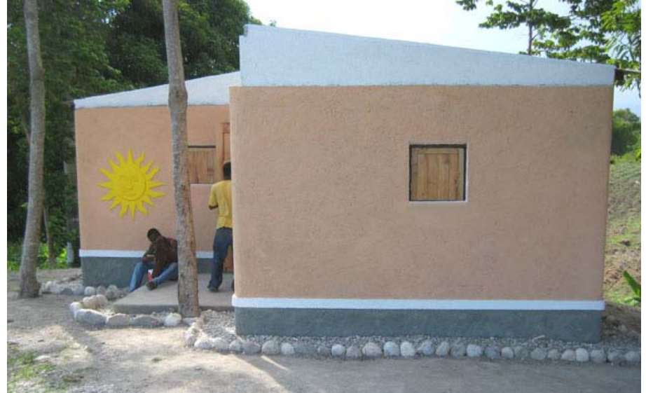
Image used with permission from www.earthbagbuilding.com
