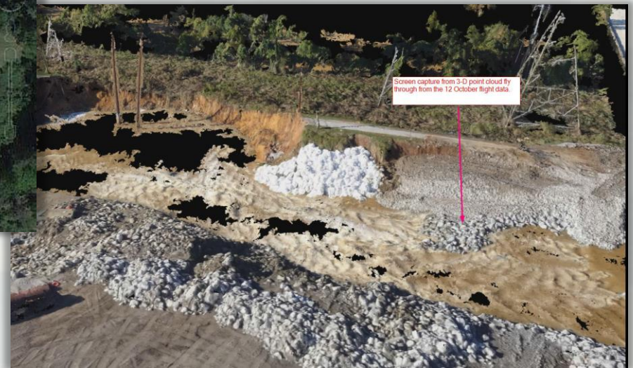
West Bank of Columbia Canal; rendered point cloud from geospatial data shown
