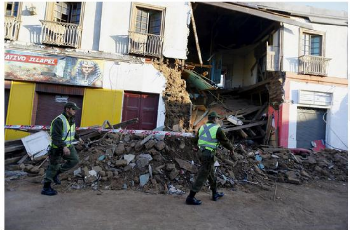
Police officers placed tape around a damaged building in Illapel, Chile, on Thursday, a day after an earthquake hit the country. Ivan Alvarado/Reuters
