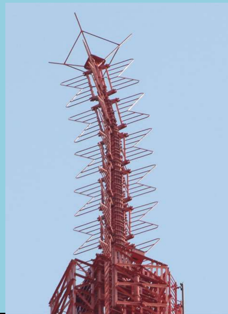
Cell tower in Tokyo after March 2011 M9
