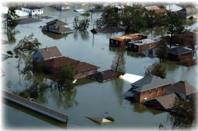
Flooding in New Orleans from Hurricane Katrina, 2005. Photograph credit: Jocelyn Augustino, Federal Emergency Management Agency; public domain.
